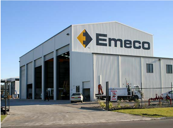
Emeco Premises – Rutherford, NSW
