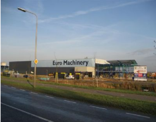
Euro Machinery New Premises – Hardenburg, Netherlands
