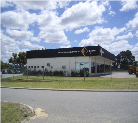
Emeco Premises - Redcliffe, WA
