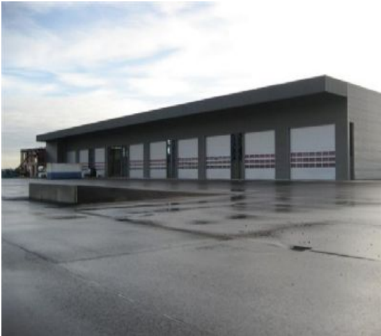
Euro Machinery New Premises – Hardenburg, Netherlands
