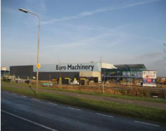
Euro Machinery New Premises – Hardenburg, Netherlands
